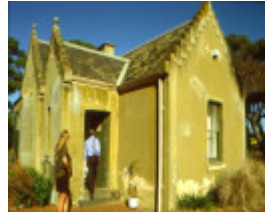
1 overnewton gatehouse h1947 march 2001
