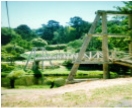
Warburton Swing Bridge
