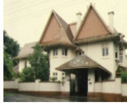
1 glyn kooyong road toorak front view
