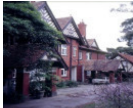
edzell st georges road toorak south facade she project 2003
