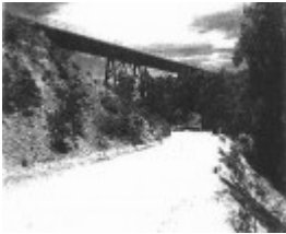
Railway Viaduct, Bridge and Embankment
