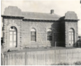
B0864 Old Shire Hall Portland
