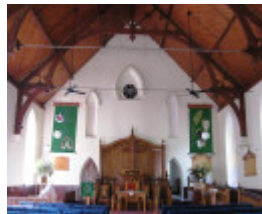
St Andrews interior
