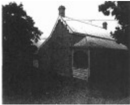
Webster Brothers yard & former "The Iron Church"
