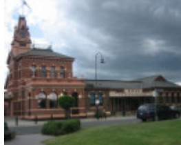
Traralgon Post Office from the north side
