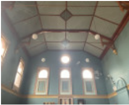
Court Room ceiling
