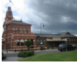
Traralgon Post Office from the north side
