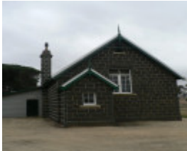
Former State School, now Public Hall, Murgheboluc
