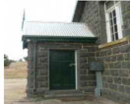
Entrance Porch, Former State School, Murgheboluc
