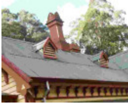
Before Photograph - Reference F3834 2014
