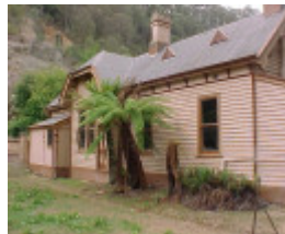
H00583 walhalla po exterior side mar 2003
