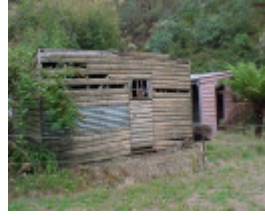
Walhalla Post Office Exterior Outbuildings March 2003
