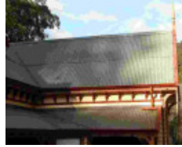
Before Photograph - Reference F3834 2014
