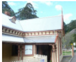
After Photograph - Reference F3834 2016
