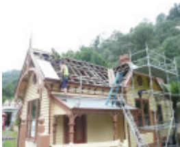
During Photograph - Reference F3834 2015
