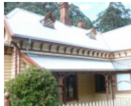
After Photograph - Reference F3834 2016
