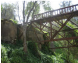
Brunton s Bridge, Walhalla end from below
