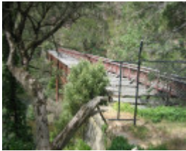
Bruntons Bridge Thompson River
