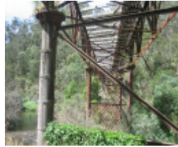
Bruntons Bridge Thompson River
