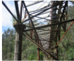
Brunton s Bridge from below
