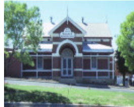
1 ovens & murray hospital for the aged warners road beechworth front view
