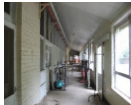
Recreation wing corridor
