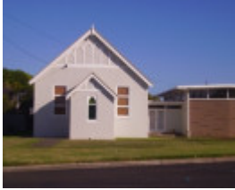
Former St Andrews Church and Hall, Dennington
