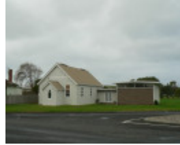
St Andrews Church and Hall (former), Dennington
