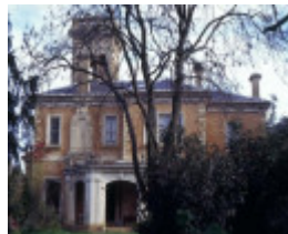
bontharambo homestead boorhaman road wangeratta garden she project 2003
