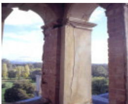
bontharambo homestead boorhaman road wangeratta view from tower she project 2003
