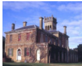
bontharambo homestead boorhaman road wangeratta back view of homestead she project 2003
