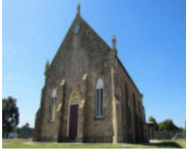
HO21 Uniting Church Old Western Highway Myrniong
