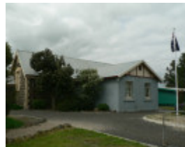
Lethbridge State School 2846 Midland Highway Lethbridge
