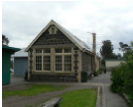
Lethbridge State School 2846 Midland Highway Lethbridge
