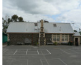
Lethbridge State School 2846 Midland Highway Lethbridge
