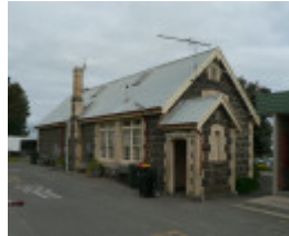
Lethbridge State School 2846 Midland Highway Lethbridge
