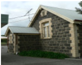
Lethbridge State School 2846 Midland Highway Lethbridge
