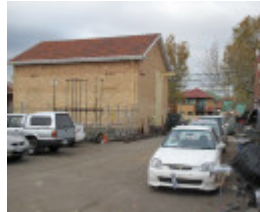
MMTB substation_Thornbury_14 May 2009_mz
