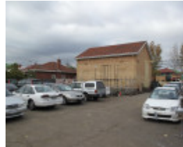
MMTB substation_Thornbury_14 May 2009_mz
