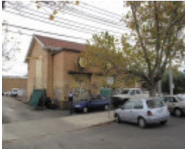
MMTB substation_Thornbury_14 May 2009_mz
