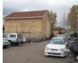
MMTB substation_Thornbury_14 May 2009_mz
