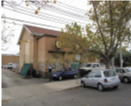
MMTB substation_Thornbury_14 May 2009_mz
