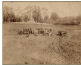
Chinamans Lagoon during construction 1878
