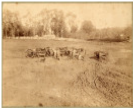
Chinamans Lagoon during construction 1878
