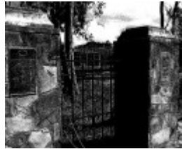
HO249 - detail of pedestrian gate
