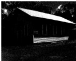
HO248 - Plenty Hall, view from south-east
