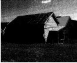
HO243 - View from south, with added new wing on north
