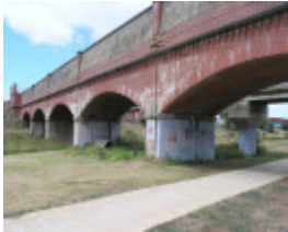
MAIN OUTFALL SEWER SOHE 2008
