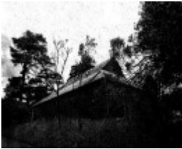
HO212 -Shaw's Cool Store & residence- Cool store, packing shed from Shaws Road
