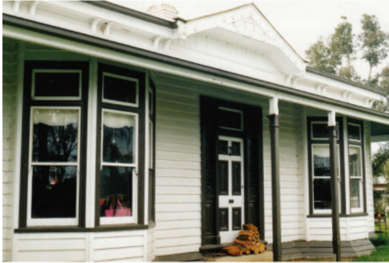
HO204 - Edendale - Eltham Pound Keepers Residence 2.jpg
