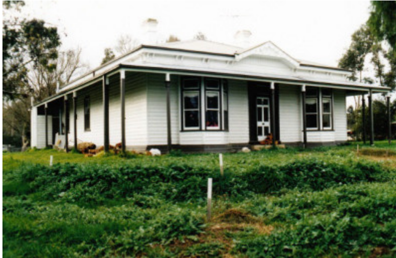
HO204 - Edendale - Eltham Pound Keepers Residence.jpg
