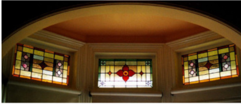
HO204 - Edendale - Eltham Pound Keepers Residence leadlighting 3.jpg
