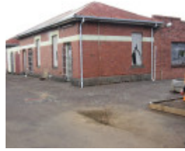
Warragul Railway Station drivers room
