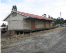
Warragul railway station goods shed from east
