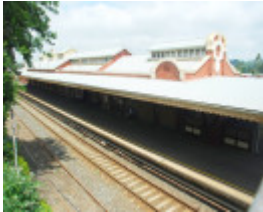
WARRAGUL RAILWAY STATION SOHE 2008
