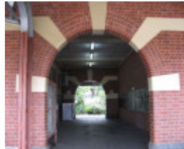
Warragul Railway Station link between 2 platforms
