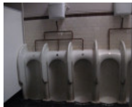
Warragul Railway Station urinals
