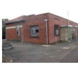
Warragul Railway Station drivers room addition
