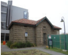
POLICE STATION COMPLEX SOHE 2008
