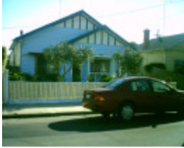
3 George Street, Geelong West
