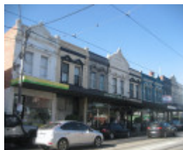
Victorian shops, 475-487 Malvern Road
