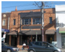
Former ES&A Bank, 510 Malvern Road
