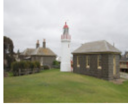
LADY BAY LIGHTHOUSE COMPLEX SOHE 2008
