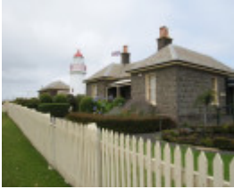
LADY BAY LIGHTHOUSE COMPLEX SOHE 2008
