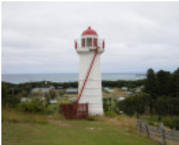
LADY BAY LIGHTHOUSE COMPLEX SOHE 2008
