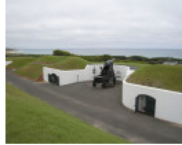
LADY BAY LIGHTHOUSE COMPLEX SOHE 2008
