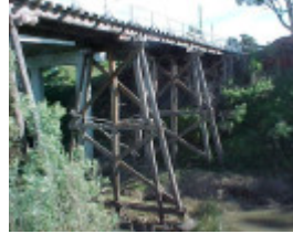
1 trestle bridge toward new bridge may01
