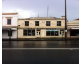
Appearance prior to repairs in 2013
