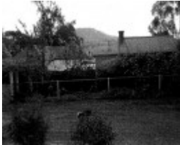
APTED FARM BUILDINGS - rear view of house with outbuildings
