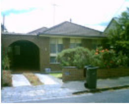
8 Plunkett Street, Geelong West
