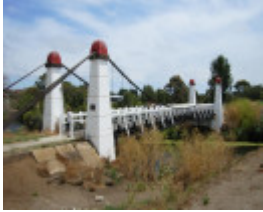
WOLLASTON BRIDGE SOHE 2008
