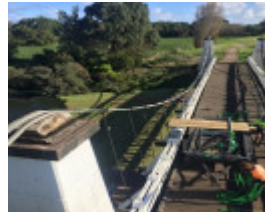
During Photograph - Reference F3855 2014
