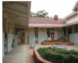
Bendigo Senior Secondary College_courtyard of 1914 building_KJ_Nov 09
