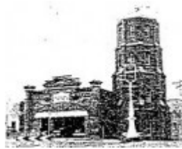
East Ballarat Fire Station - Ballarat Conservation Study, 1978
