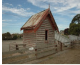
Former Caretaker's Cottage, west elevation
