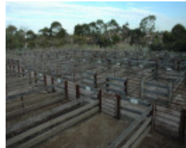
Overview of sheep pens showing introduced steel posts (former tram tracks) and horizontal timber rail.
