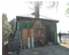
Market Offices building, south elevation
