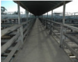
Details of covered way looking west.
