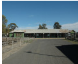
Market office buildings, east elevation
