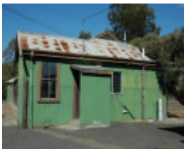
Market Offices building, north elevation
