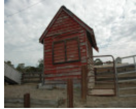
Former Caretaker's Cottage, east elevation
