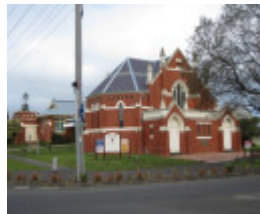
St Andrews Uniting Church and church hall
