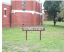
St Andrews Uniting Church and church hall
