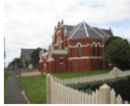
St Andrews Uniting Church and church hall
