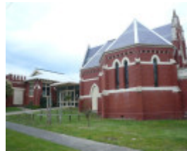
St Andrews Uniting Church and church hall
