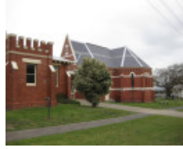
St Andrews Uniting Church and church hall
