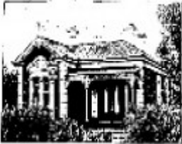
Residence 504 Darling St - Ballarat Conservation Study, 1978
