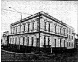
Ballarat City Council Offices - Ballarat Heritage Review, 1998
