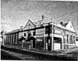
Offices Sunnyside Mills - Ballarat Heritage Review, 1998
