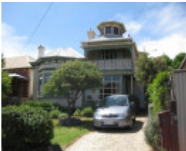
50 King Street, Queenscliff
