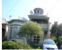
50 King Street, Queenscliff
