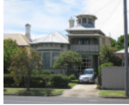
50 King Street, Queenscliff
