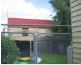
Stables 43 Carlisle Street
