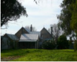
Evandale, 15-17 Stevens Street, Queenscliff
