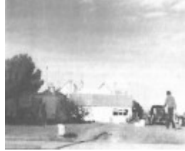
The rear west elevation of Evandale from Stevens Street., 15-17 Stevens Street, Queenscliff
