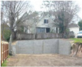
Evandale, 15-17 Stevens Street, Queenscliff
