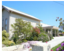
Parish/Church Hall (formerly housing the St Aloysius Primary School)
