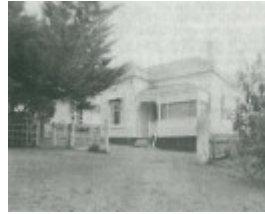
Whitby House, 8 Baillieu Street, Point Lonsdale
