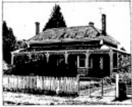
North View Villa - Ballarat Conservation Study, 1978
