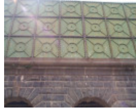
H01416 water tank werribee3 feb2003
