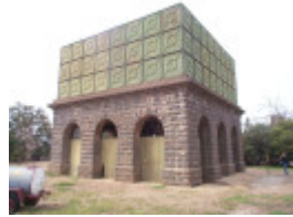
H01416 1 water tank werribee4 feb2003
