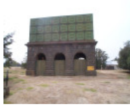
H01416 water tank werribee feb2003
