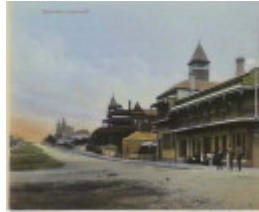
View south along Gellibrand Street c 1906 Source: SLV (a02758)
